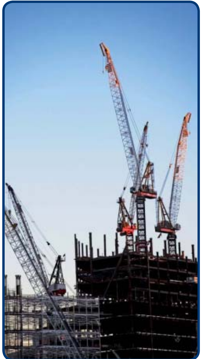
New developments require new connections to our network
