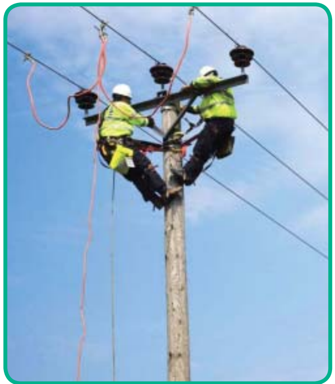
Our engineers at work replacing overhead cables
