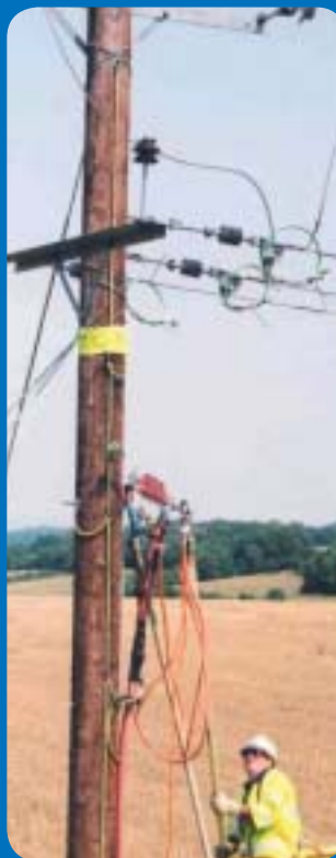
One of our engineers at work maintaining your network
