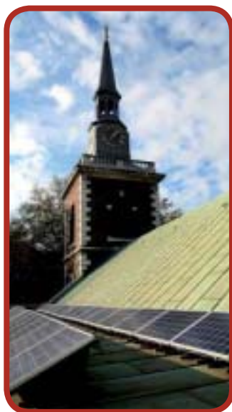
An example of local power generation on a church roof
