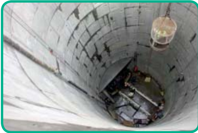
We have now installed the underground cable tunnels that will deliver power for the 2012 Olympics
