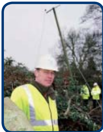
Damage caused by a storm in 2007 being inspected by EDF Energy's CEO, Vincent de Rivaz
