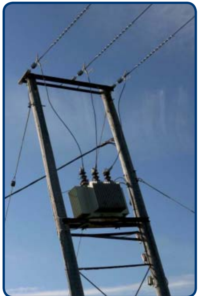
An electrical transformer
