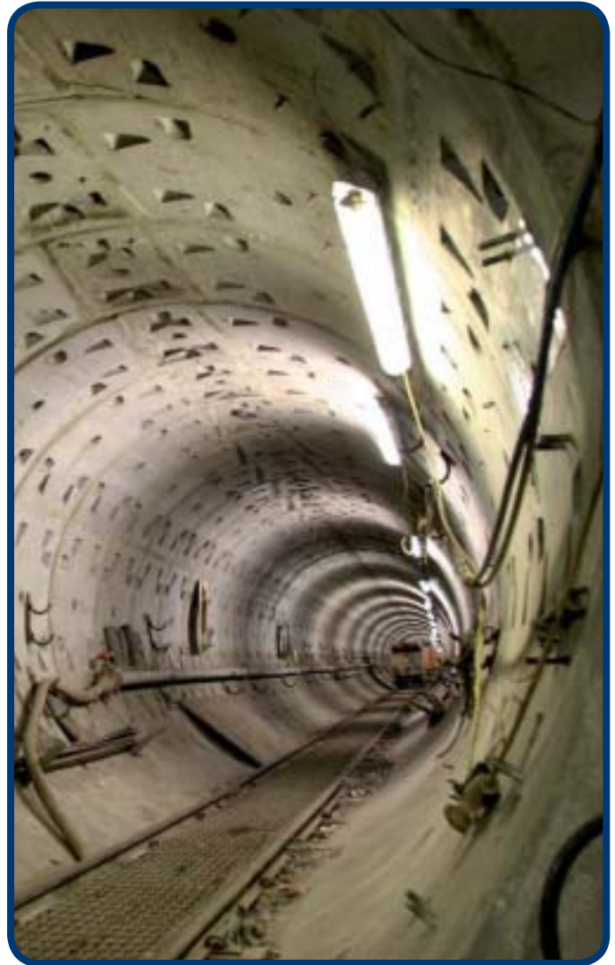
Our underground Bankside tunnel
