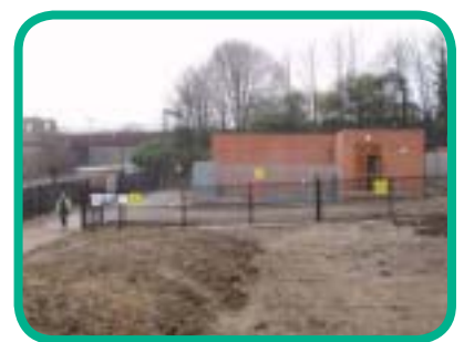
Waterside primary substation
