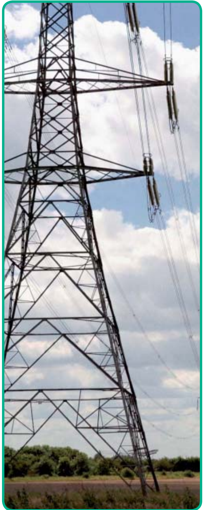
One of our electricity pylons, delivering power to you
