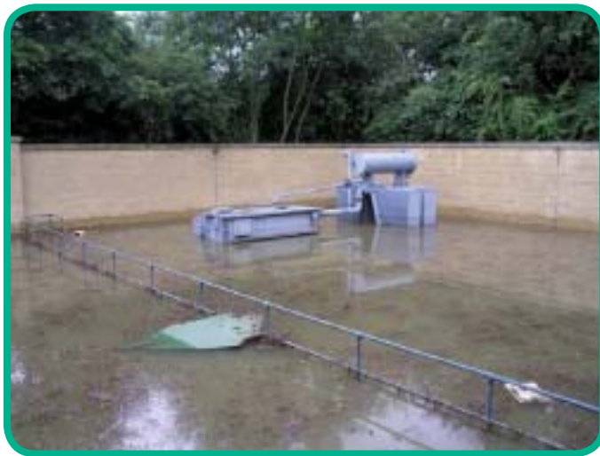
Localised flooding of EDF Energy Networks equipment at our Hemel Hempstead site
