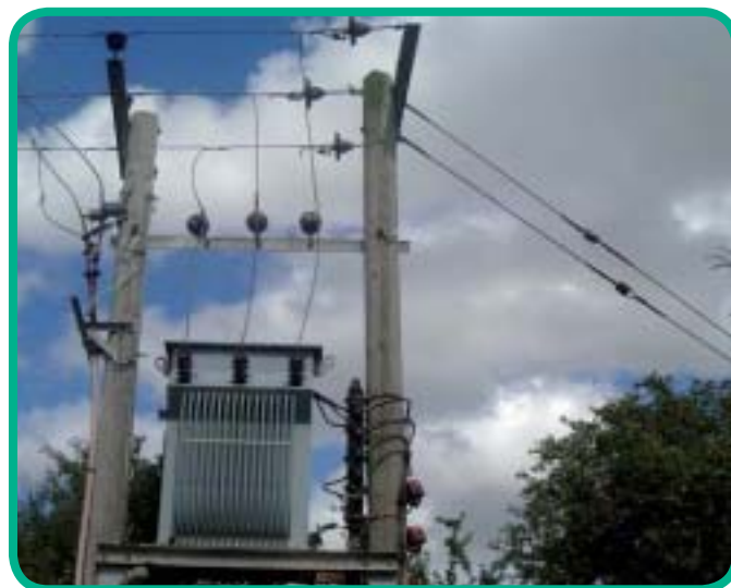
An overhead transformer, one of our many network assets
