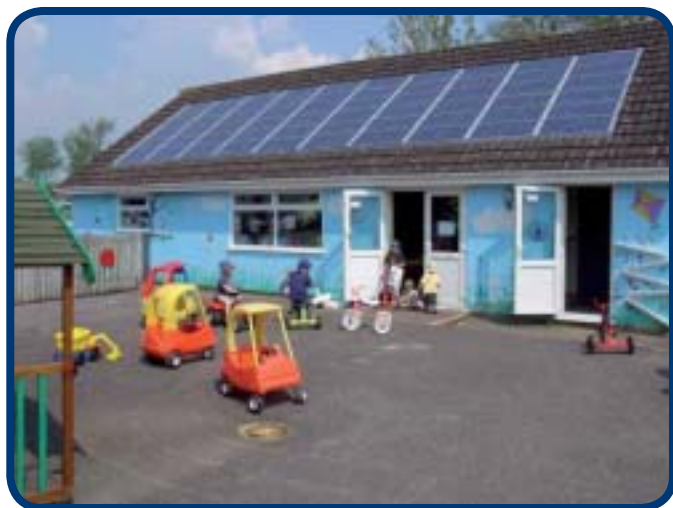
Solar panels at a pre-school, an example of renewable distributed generation
