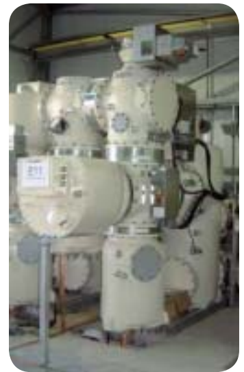
132kV substation with equipment filled with SF_6
