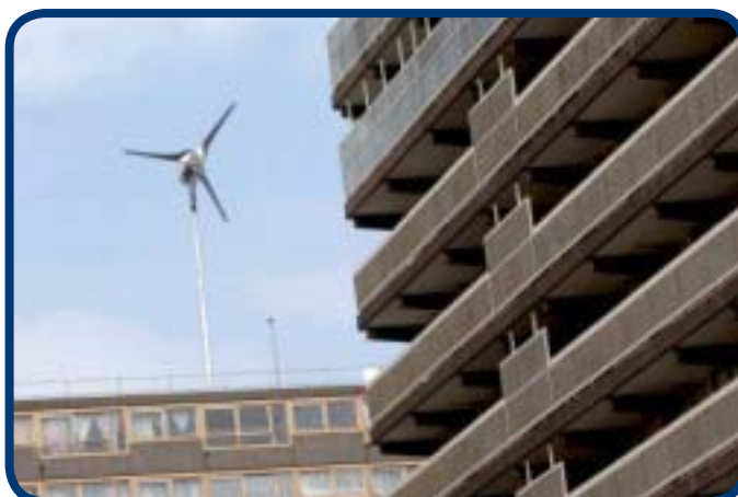
The first wind turbine to be fitted to a block of flats in Southwark, South London
