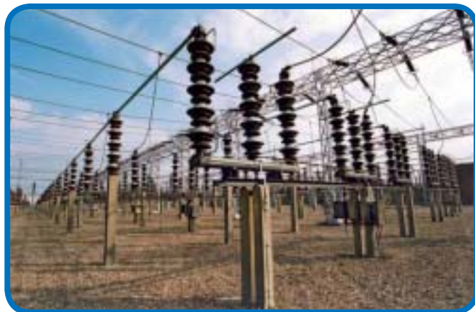
Beddington grid - an example of our grid assets
